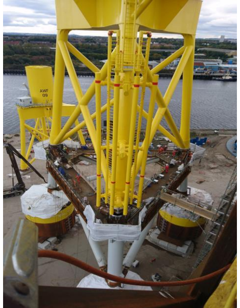
Suction Bucket Jacket Foundation being assembled in Newcastle.
